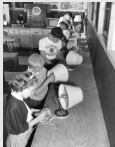
4-H electric project, mid-1900s
